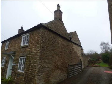
General view of west elevation looking up toward neighbour's drive and garden. Note ground level rises against applicant's property
