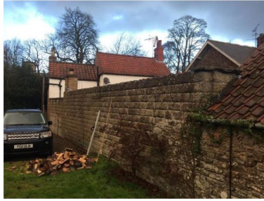
General view of existing wall to applicant's property which is constructed from coursed modern concrete stone effect blocks.
